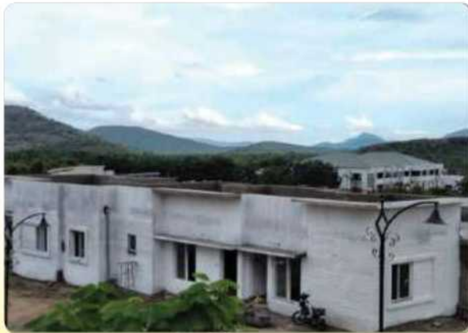
Villas Under Construction at Site
